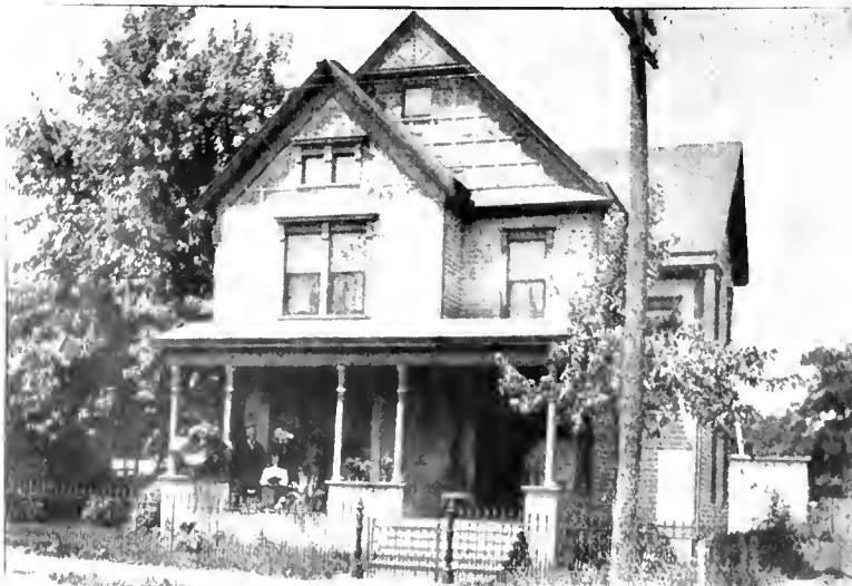
RESIDENCE OF PROF. J. D. COLLINS. South 5th Street.
